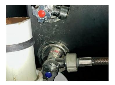
Another tap that might fail is the washing machine hot water tap located in the laundry cupboard under the sink. This hot water tap should also be capped-off if not used or connected to your washing machine. For example, some washing machines only draw cold water (and then heat the water if needed).
